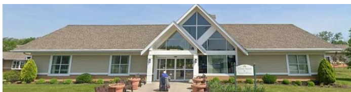
Unity-Village Community Center in Greece
